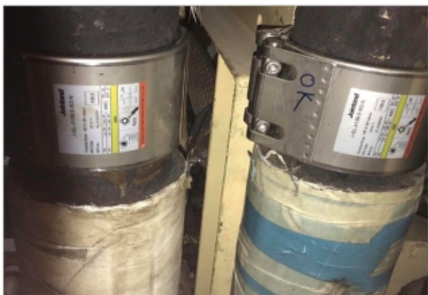
For Kd Pahang periodic repair ,Jointand pipe joint for connection was used in oil and water systems.
