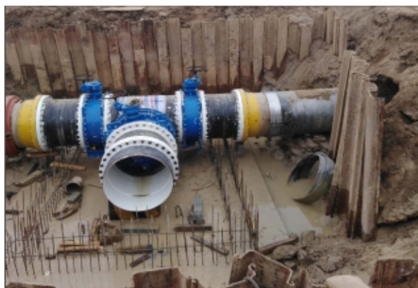
The newly built water conveyance project of Xiamen Water uses Jointand FLEX pipe joint for connection, eliminating traditional complicated construction mode.
