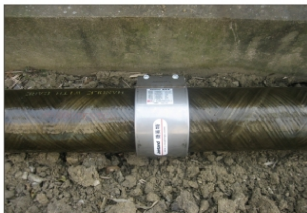
Glass fiber reinforced plastic pipe uses Jointand FLEX pipe joint for connection, and saves flange and other complicated construction modes
