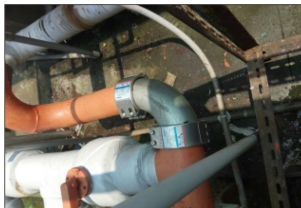
The air-conditioning cooling water pipe uses Jointand pipe joint, eliminating the traditional welding procedure method.
