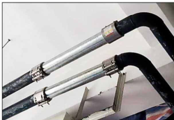
Pipeline reconstruction of water system of high-rise buildings uses Jointand pipe joint for connection.
