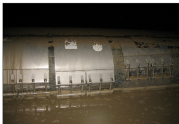
Xiamen Water uses Jointand dual-phase stainless steel pipe joint for rush repair for AD850mmHDPE pipe damage.
