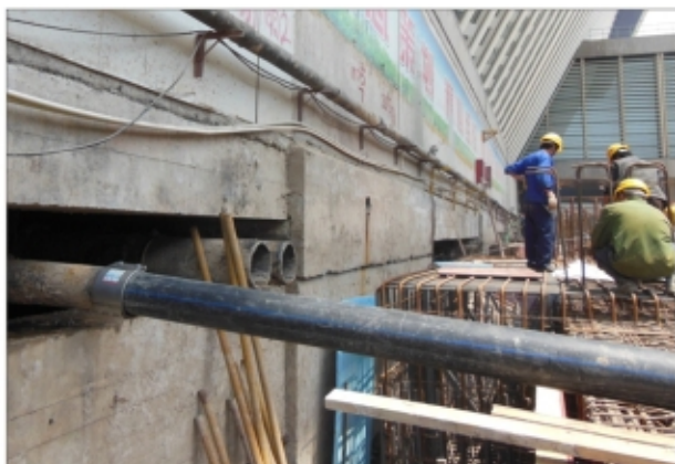
Connection of metal pipe and HDPE pipe for Shanghai Pudong Airport T1 terminal expansion uses Jointand pipe joint.
