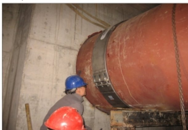
Wuhan Tap Water AD1620mm welding steel pipe uses Jointand FLEX pipe joint.
